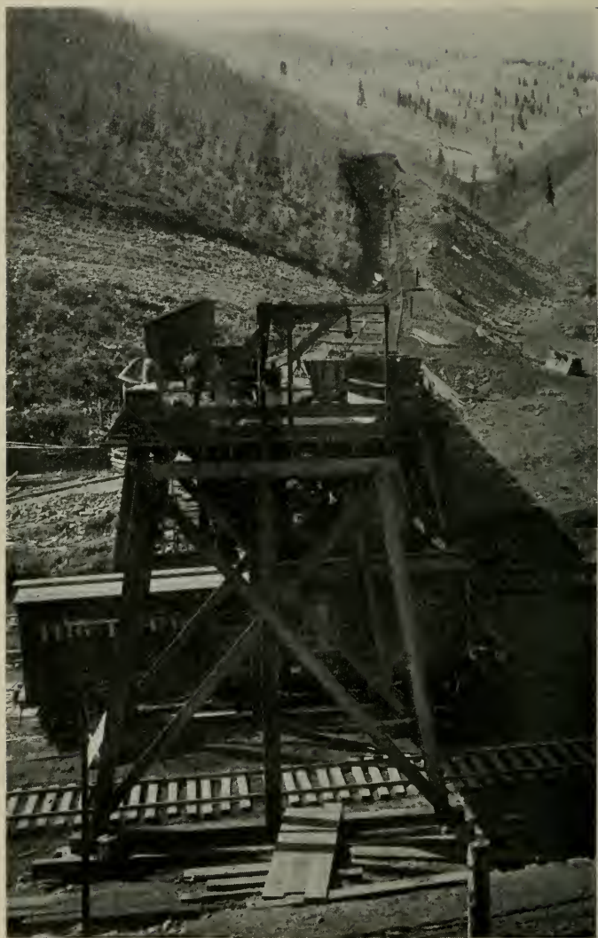
Trestle, Dump and Incline of No. Four Mine.
